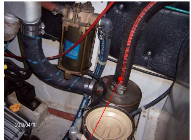
B4 exhaust hose is fuel fill hose not suitable for use as exhaust hose
