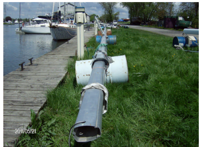
mast as inspected
