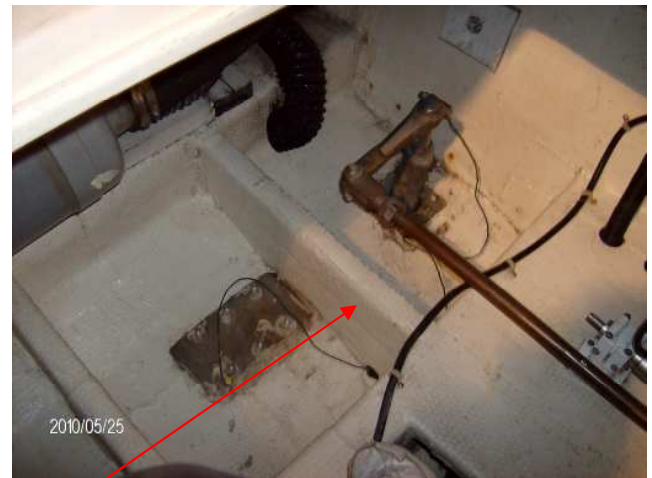
C2 Delamination suggested here Bilge is free of oil contamination
